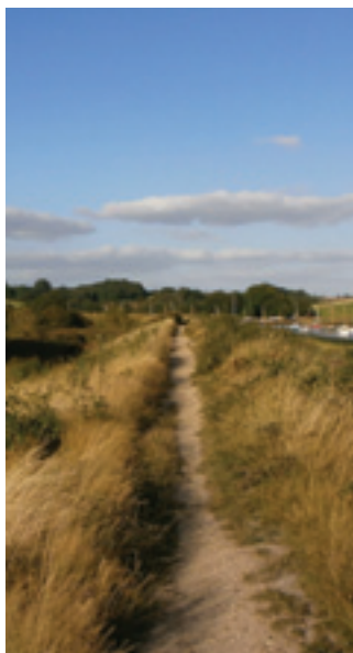
△ Sea wall crest
