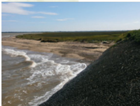
▽ Open stone asphalt revetment on a sea wall
